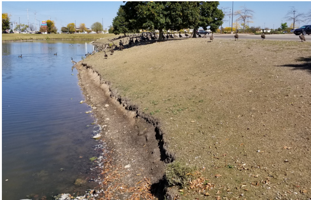
Turf Grass Pond - Severe shoreline erosion
