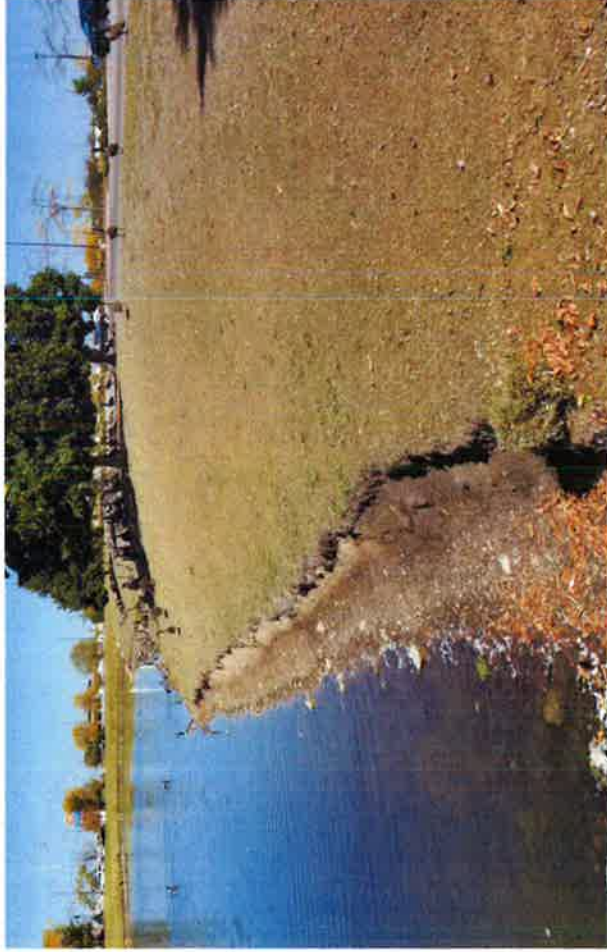
Turf Grass Pond - Severe shoreline erosion
