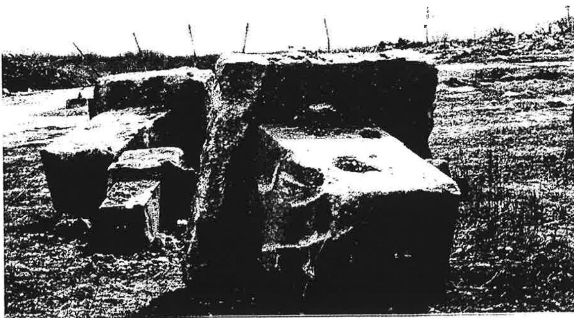
Typical foundation for above ground piping support column.
